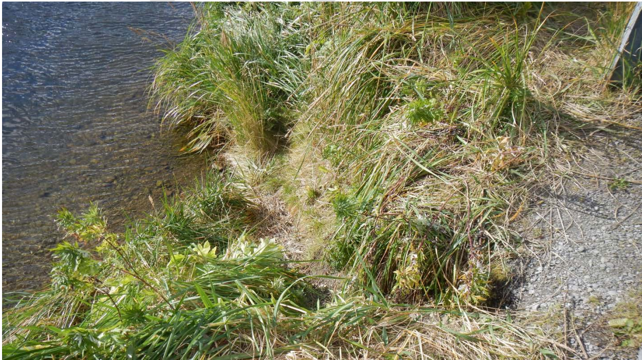
Photo 2-3. Noted Erosion along the Banks of the Lower Iliuliuk River due to Foot Traffic
