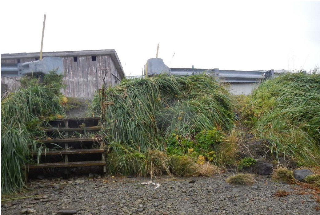
Picture 1. River access stairs and impacted vegetation area.
