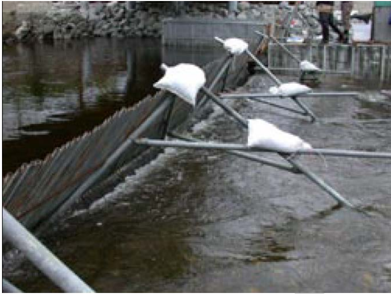
Photo 3-4. Rigid Tripod Weir Example (Zimmerman & Zabkar)
