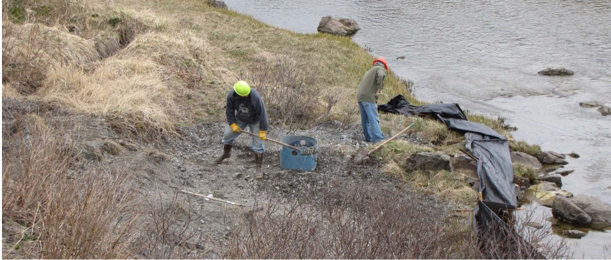
Photo 2-5. City Roads Crews Cleaning up Snow Dump along South Bank of the River
