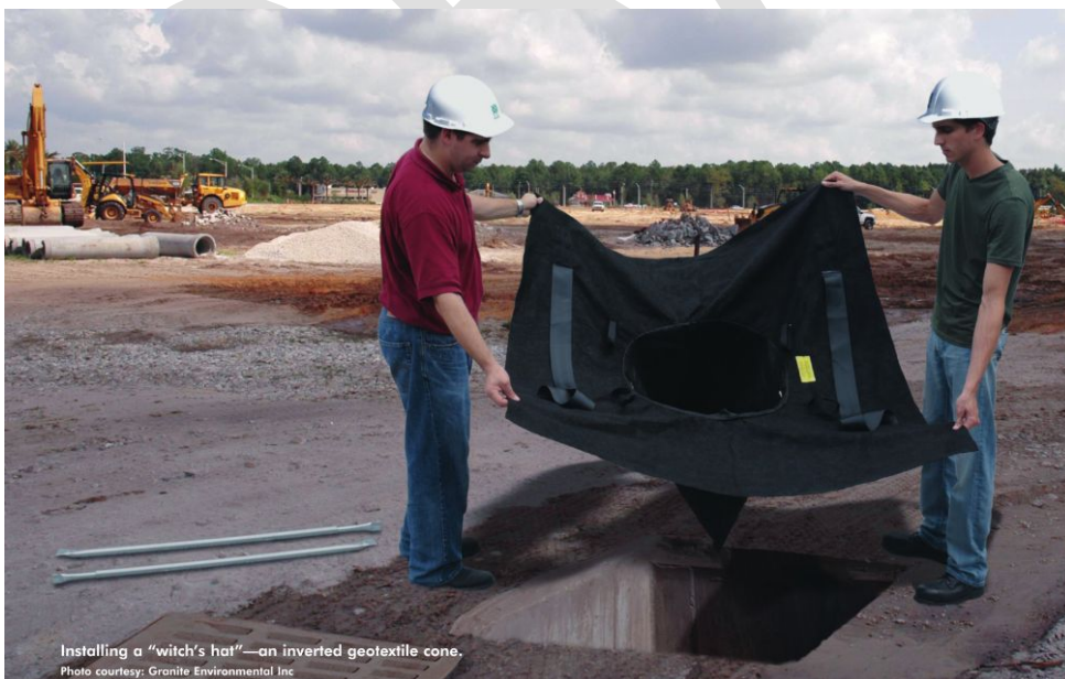
Figure 6-1. Witch's Hat Installation (Williams-Villano 2013)
