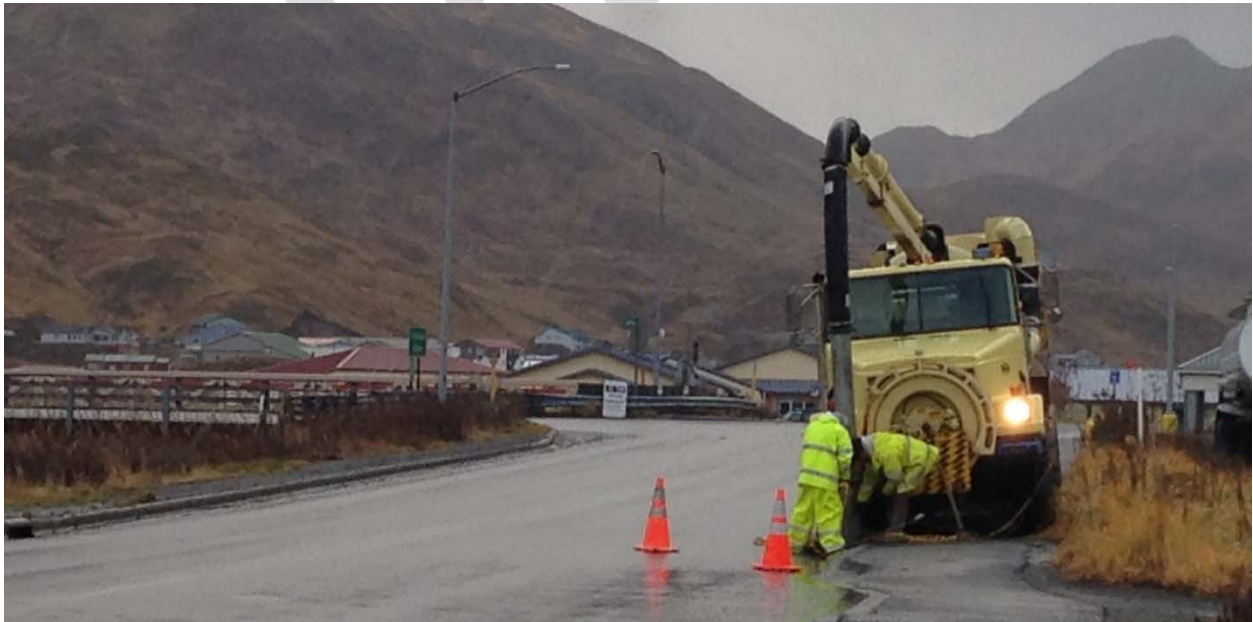
Photo 8-3. City Cleaning Storm Drain with a Vacuum Truck
