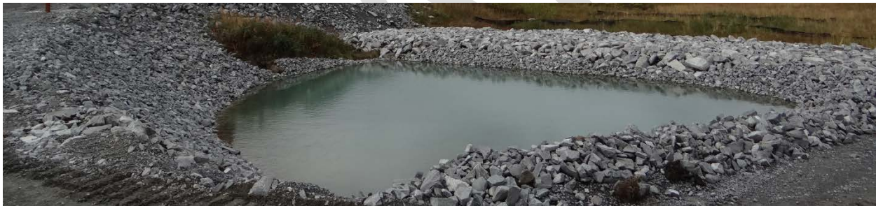
Photo 6-2. Sediment Basin at Ugadega Quarry
