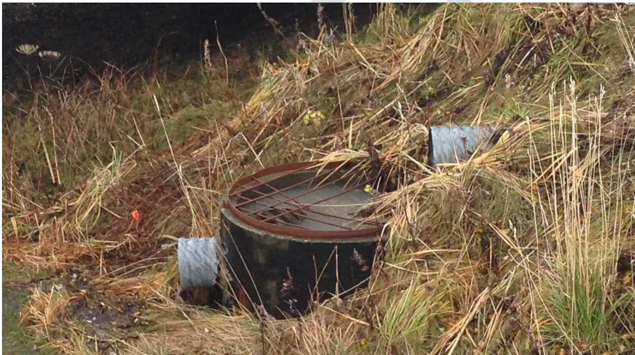
Photo 8-5. Engineered Outfall at 5th Street Bridge
