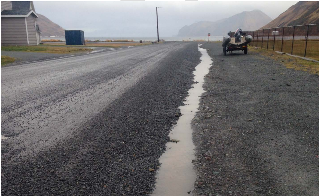
Photo 8-9. Sediment-Laden Runoff in King Street Ditch (looking northeast from Duck Pond Lot)
